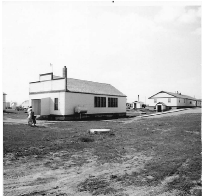
Spring Creek's Church/School House and Kitchen/Dining Hall.
